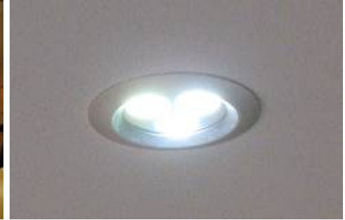
Fig 3: Close up – LED down lighter
